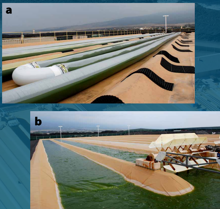
FIGURE B1. The Cellana Kona Demonstration Facility (KDF) where demonstration-scale cultivation experiments using ALDUO™ technology were conducted. (a) Closed-loop photobioreactors. (b) Open raceway ponds.
