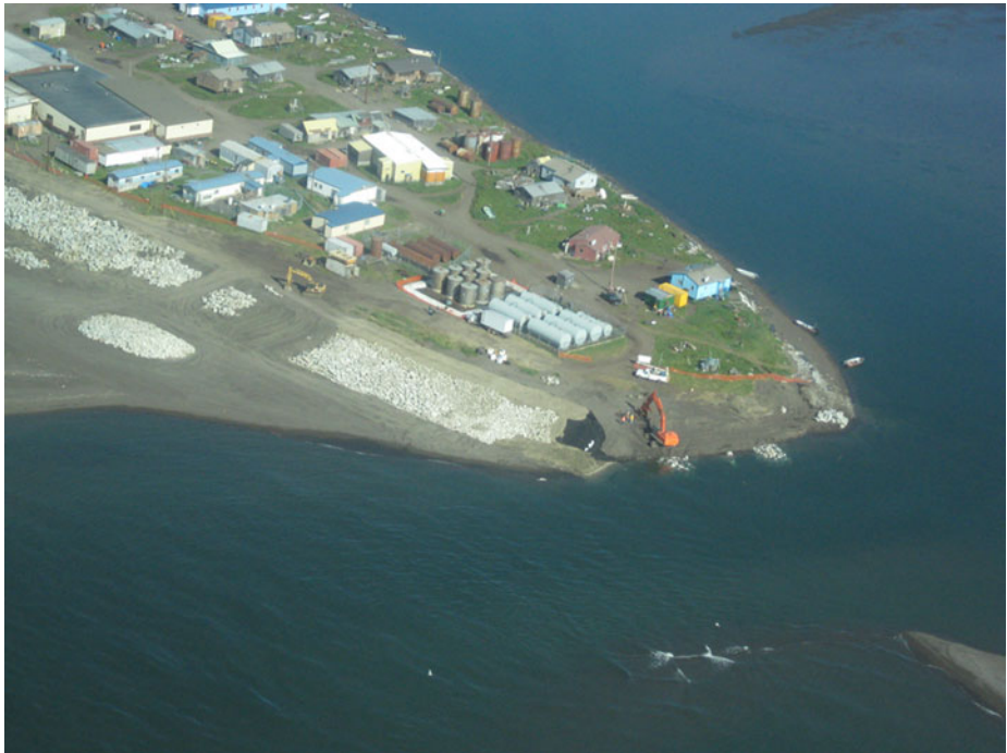
Rock revetment project under construction, Kivalina 2008. Source: Christine Shearer
