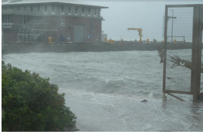
Wave overtopping at Waterfront Park
