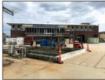
Climate Vulnerability Assessment – Asset Profile
