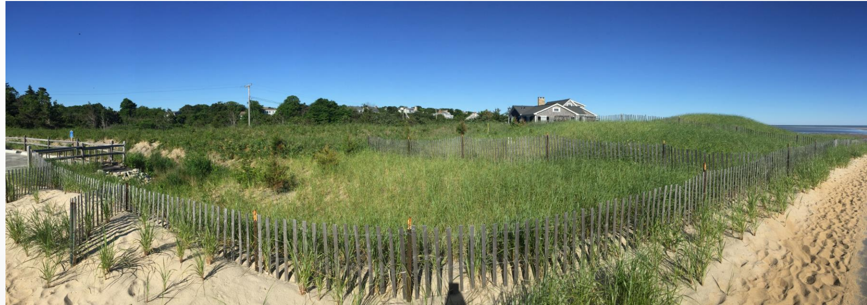
Dune reconstruction at previously flooded and eroded coastal parking lot (Breakwater Beach, Brewster)
