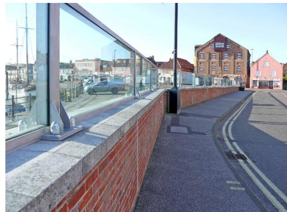
Glass flood walls using structural glass preserve views and can be installed atop existing walls or on their own; floodproof windows are also available ( https://floodcontrolinternational.com )
