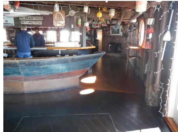
The Landfall Restaurant has integrated a range of wet floodproofing measures over the years, including removable glass doors, a floodable dining area with pop out floor hatches to relieve wave pressure under the section on piers, and a breakaway rear wall
