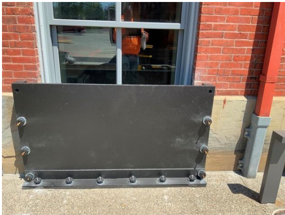
Barrier panels can be installed on door and windows, and typically have a gasket to make the seal to wall and ground. Some products can be linked together with posts to form a fence-like barrier linked to, or independent of, the building ( floodriskamerica.com )
