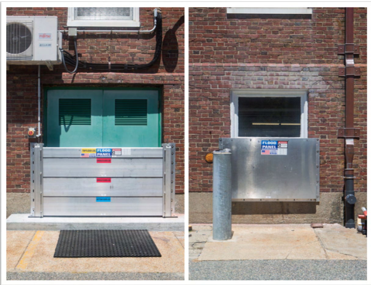
Figure 14. Bigelow deployable barrier installation on key windows and door.
