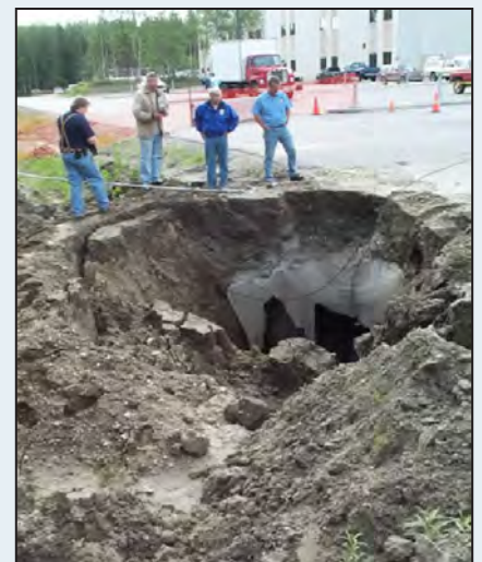
Figure 14: Thermokarst depression on the edge of the Geophysical Institute University of Alaska Fairbanks parking lot (Fairbanks, Alaska). Surface disturbance related to the parking lot construction triggered permafrost degradation and ground ice melting. From: http://www.arctic.noaa.gov/essay_romanovsky.html Photo: V. Romanovsky
